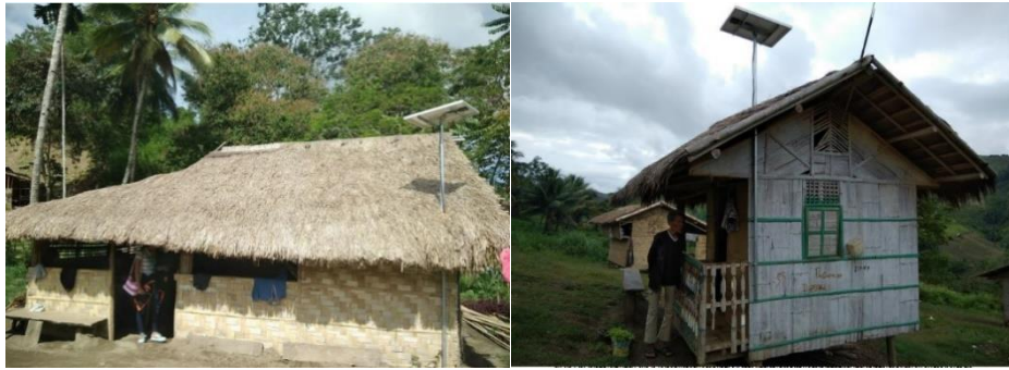
Diagram 8 : Roof-through Pole mounted installations on thatched roof
