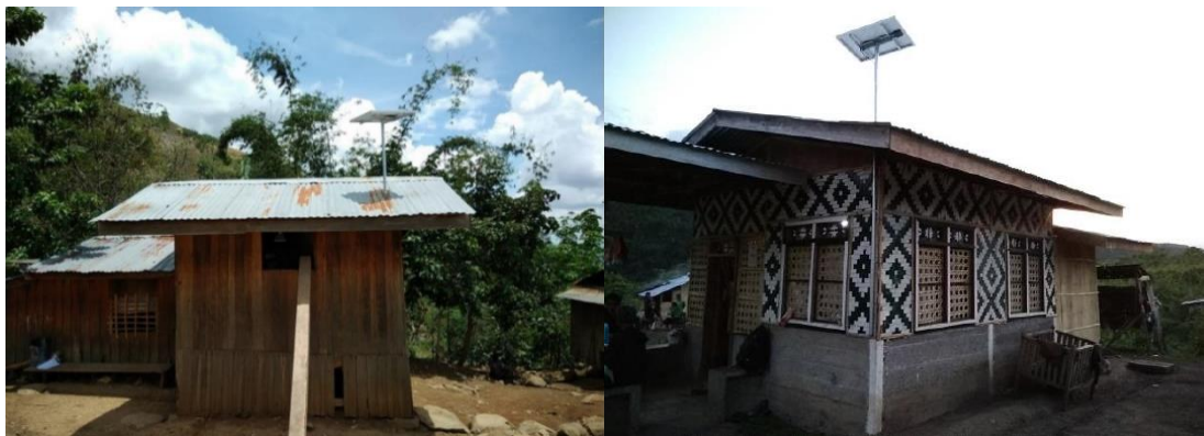
Diagram 7 : Roof-through Pole mounted installations on GI roofs
